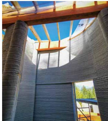
Retaining walls consist of a concrete mix that is squeezed from a nozzle and printed in layers
